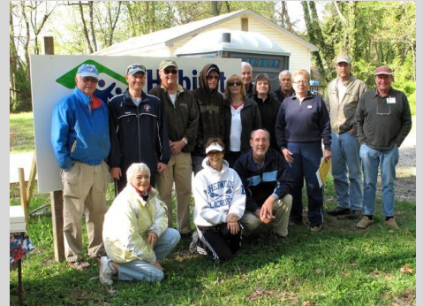
Some of our parish volunteers at the groundbreaking of the St. Michaels Faith Build on April 10, 2010.
